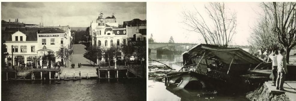
Figure 14 – Left: Frontal view of the old quay, before the earthquake, showing some 3 m from water level to top of quay. Right: After the earthquake, the collapsed quay and the apparent raised water level.
