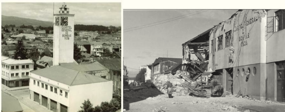
Figure 3 –Main Fire Station, at the nearby of Plaza de la República. Reinforced Concrete construction (1936). Before and after the earthquake, with the reinforced concrete tower collapsed over the street.
