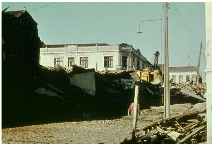
Figure 2 – An hybrid construction at the left (UACH photo) (heavy ornate façade over wood building). Right: Total destruction after the quake in a rear view. Note the great deal of contrast with the background undamaged constructions, made out solely of wood
