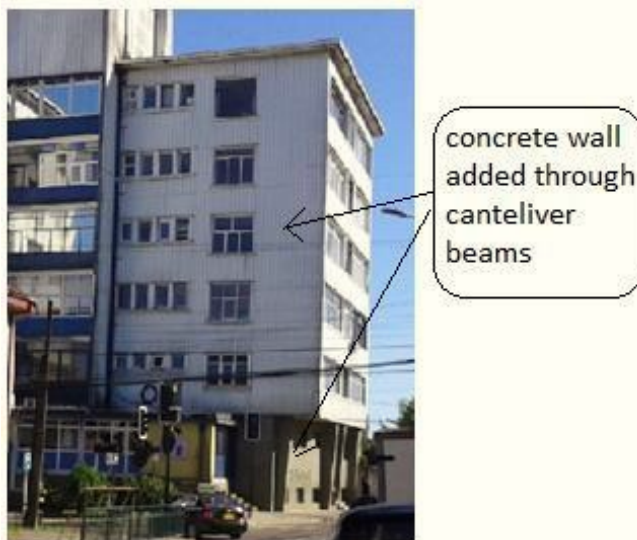
Figure - 11 The recovered building nowadays
