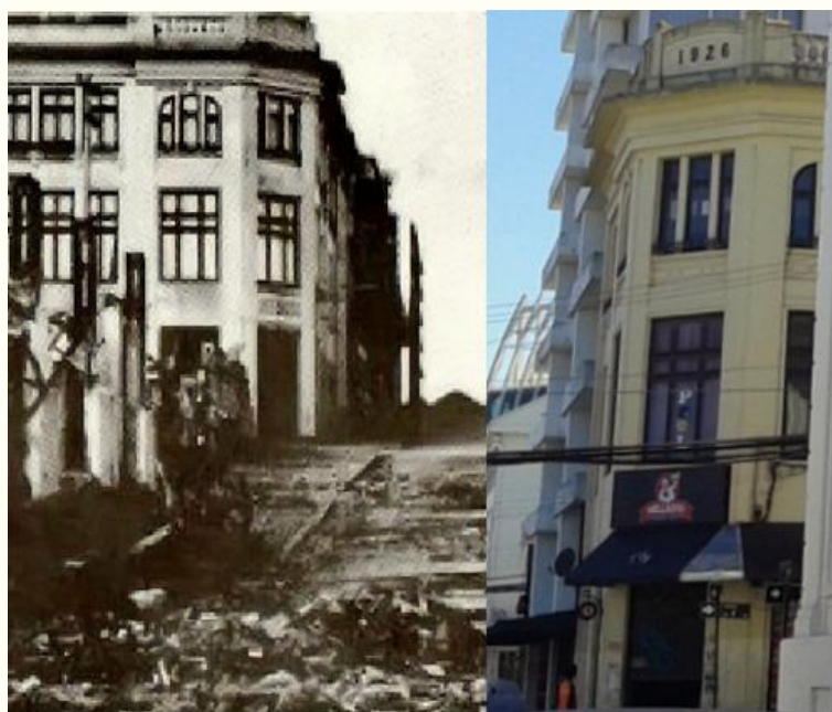
Figure 6 – A good example of endurance in a building from the beginning of XX century. On the left, after the earthquake, in the foreground are the remains of a composite steel-concrete construction. Apparently, some demolition works would have started, since that degree of destruction was not common for that type of building. At the corner in the background, an undamaged RC building from 1926. This building has been preserved in good shape up to the present day (color picture on the right). It is provided with sound concrete walls all along the back sides and all the rest is made up of RC frames. Certainly, the good result is showing also construction quality and remarkable workmanship.
