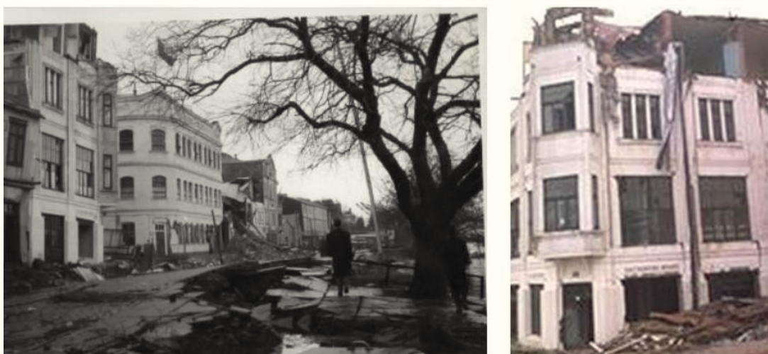
Figure 5 – Same buildings as above, showing also destruction of the quay after the earthquake. Both buildings on the corner were composite steel-concrete construction. They suffered severe damage and were demolished. Despite they were settled in very bad soil [3], the pattern of damage seemingly did not reflect a governing foundation failure. In fact, after demolition, their supporting piles came into sight in good standing, including steel ties, in between.
