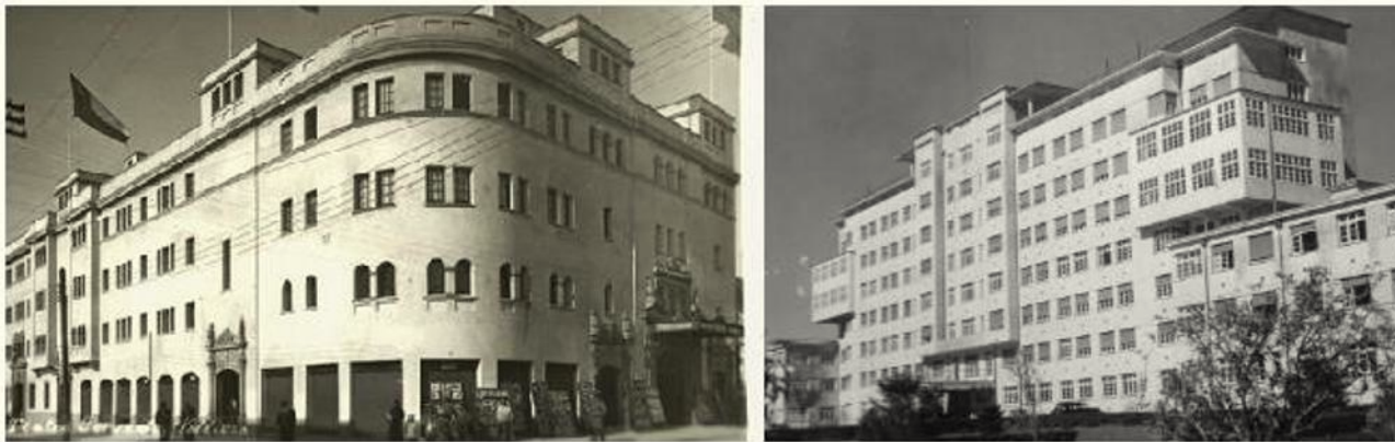
Figure 7 – Two different buildings from the late 30s. Left: Cervantes Building, built by 1935. Right: the building of Regional Hospital (postcard). This hospital was fully occupied during the earthquake and suffered serious structural damage that led to demolition. Soil conditions were fairly good in both cases, somewhat better at the site of Cervantes Building [3].
